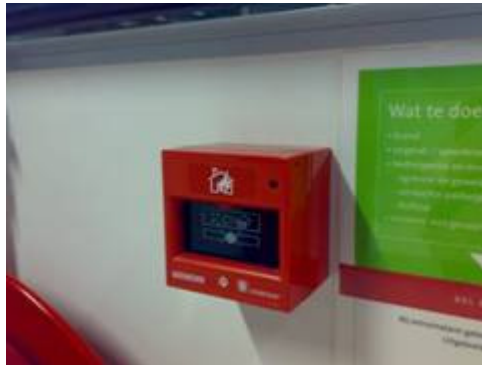
Figure 5. Manual fire alarm
